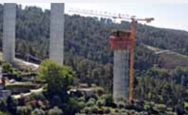
Potain-Krane errichten Pylone.
