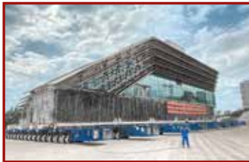
5 Sinotrans Heavy-Lift Co./TII Scheuerle
